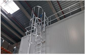
A ladder designed with safety features to prevent accidents or falls when ascending or descending from the deck.
